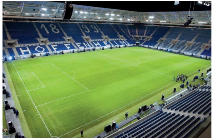
The roof structure of the football stadium belonging to TSG 1899 Hoffenheim mounted using GEDORE cordless torque wrenches.
