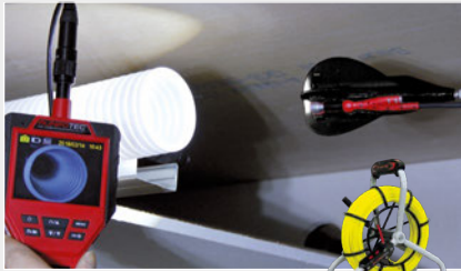
Ventilation inspection and servicing
