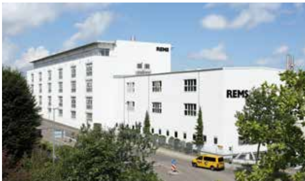
REMS training centre in Waiblingen near Stuttgart.
